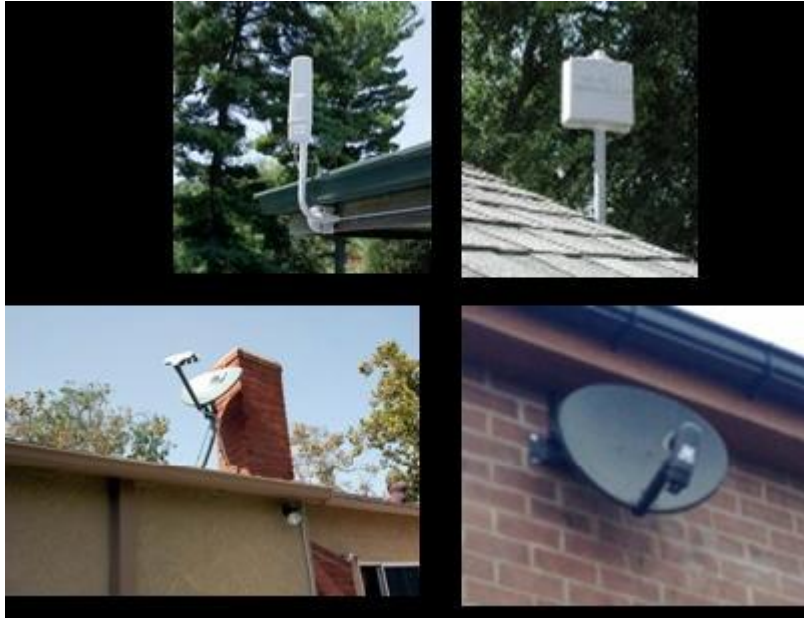
Above: examples of fixed wireless antennas (top) and satellite dishes.
